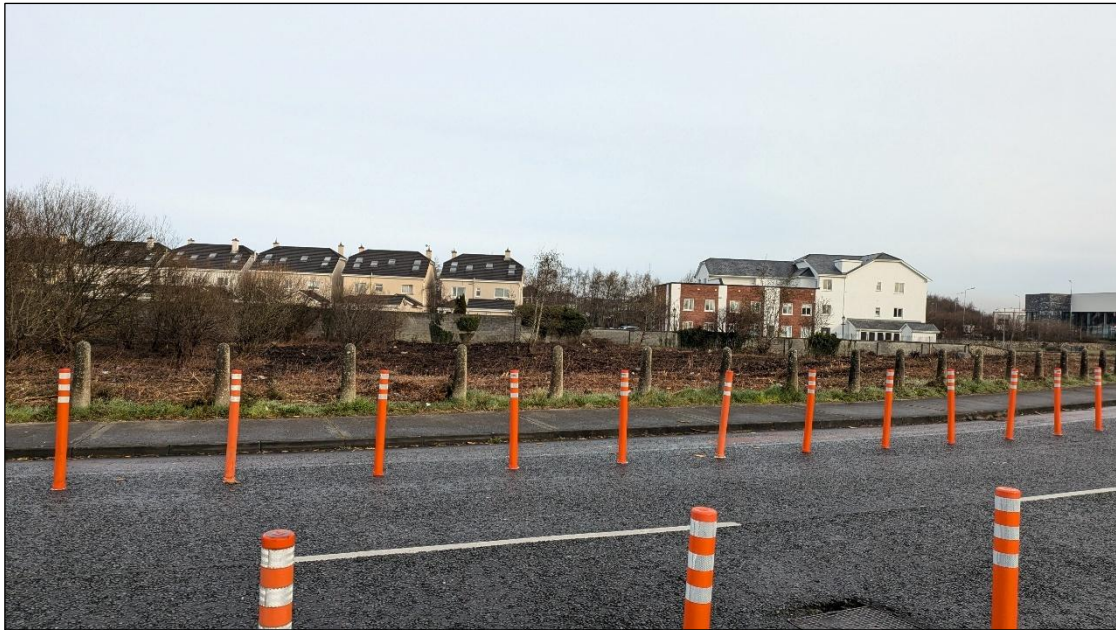
Plate 5-5 Tarmacked road (BL3) running through the site
